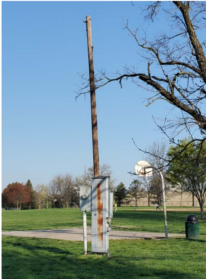
Figure 14 – Removed Light and Wiring
